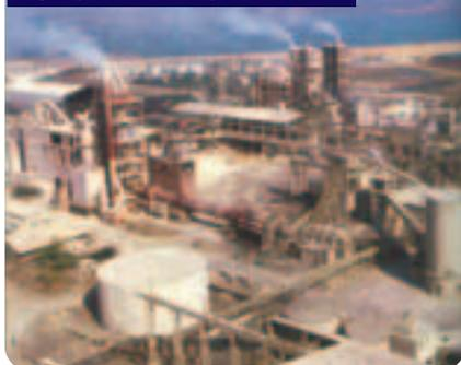
the excess heat from the clinker coolers and feeds it over all the factory and also to the surrounding residential accommodation some 2km away via insulated pipes. The boiler houses are not needed except during kiln shutdown.
